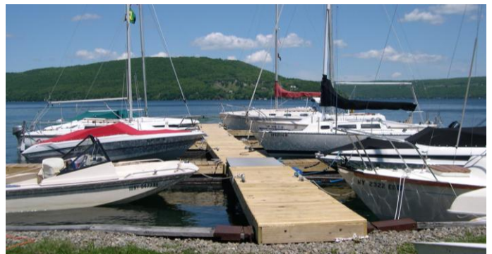
Rebuilt Floating Dock
